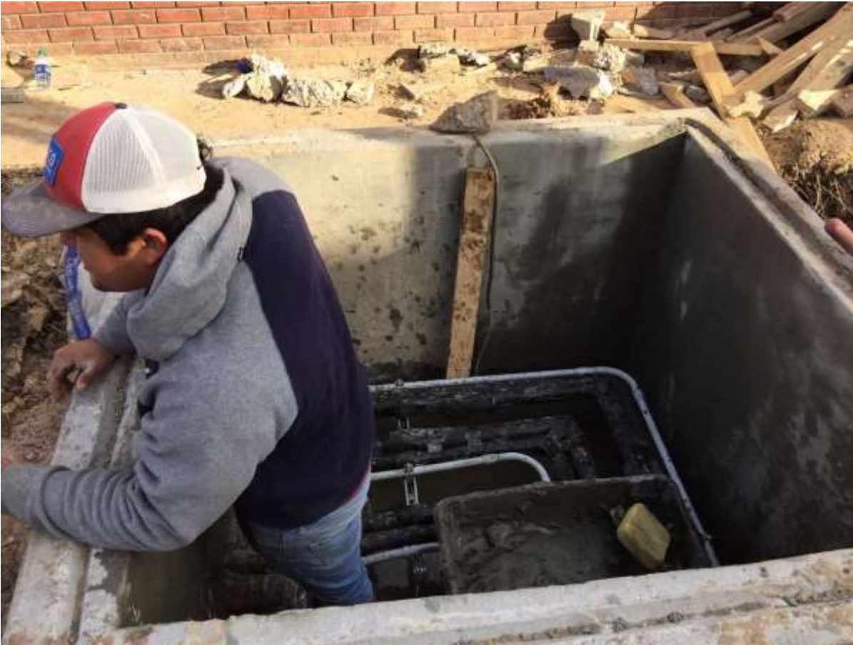
The piping and electrical conduits for the HVAC are now buried
