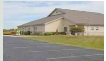
Parish Activity Center and Parish Office 670 W. Main Street Plain City, OH 43064
