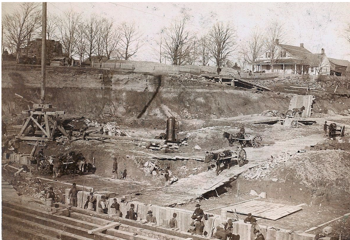
Construction of the Cornwall Canal—1897
